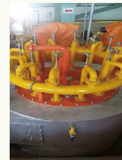
Installation of ultra-low NOx burner in Busan City Gas
