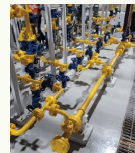
Regular inspection of facilities that handle chemicals
